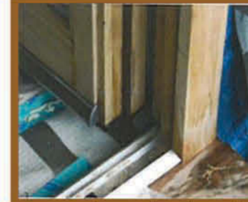
joinery, insulation and weatherproofing
