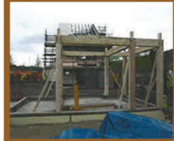
foundations, delivery & assembly of frame
