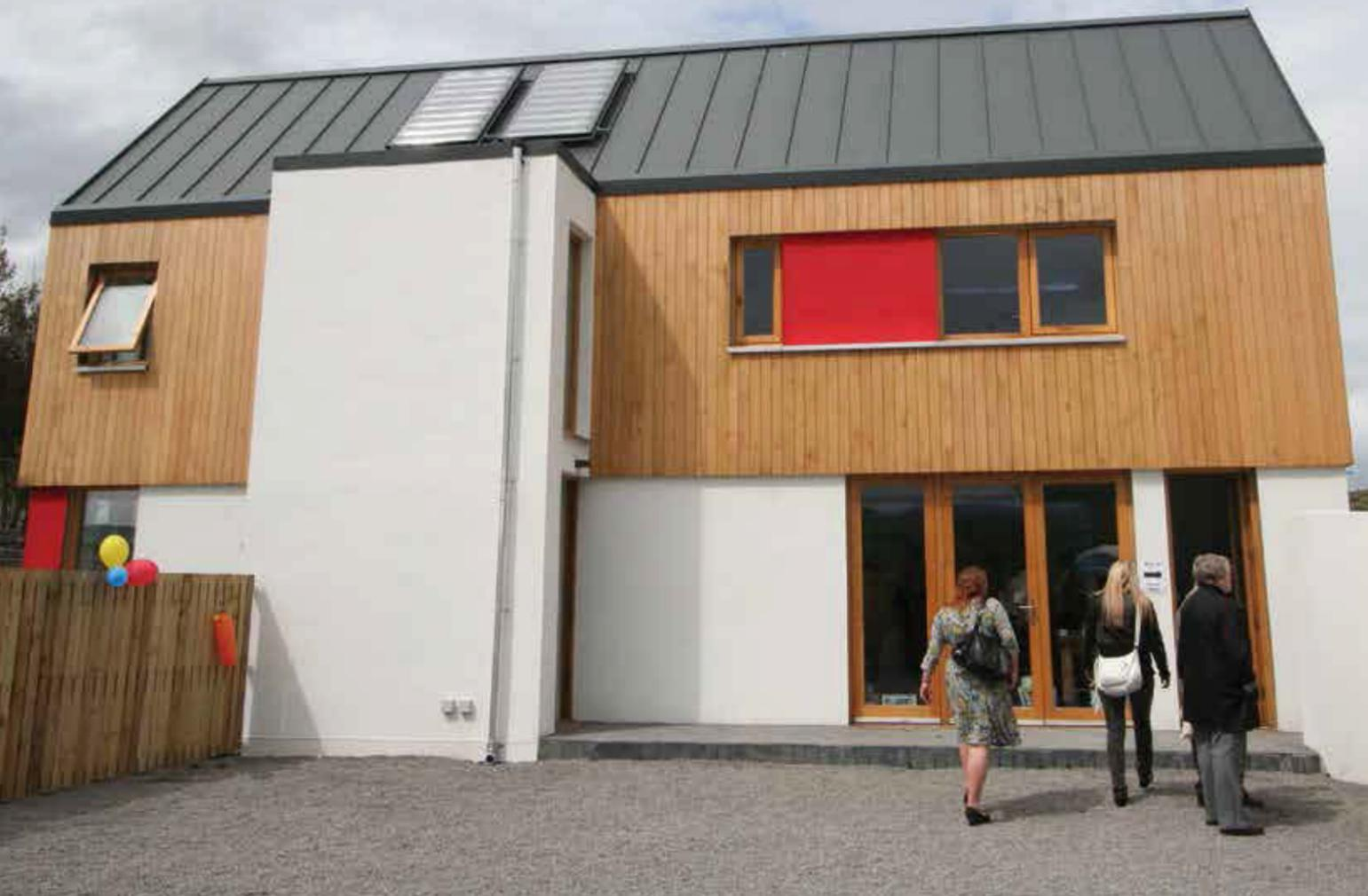
approximately 3m and can be arranged in a variety of configurations to give different building sizes and shapes. The Tŷ Unnos system is formed from two principal components; box beams and ladder beams. In addition to these standard timber joists, plywood or OSB (Oriented Strand Board) sheathing and connections are used.
