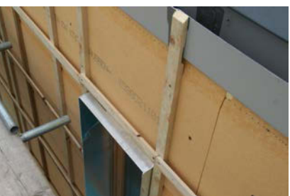
Construction detail photographs highlighting raised ground floor slab, post and beam connectors and the layered envelope to improve thermal performance
