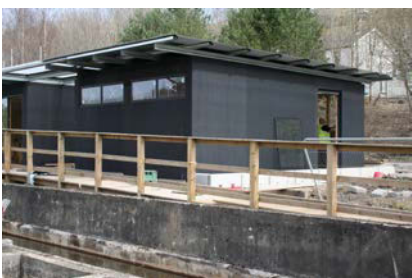
Construction sequence of the ERC, highlighting the layered and additive approach to construction, from site, to off-site fabrication and erection of box section frame and exposed SIPs infill panels for floor, walls and roof.
