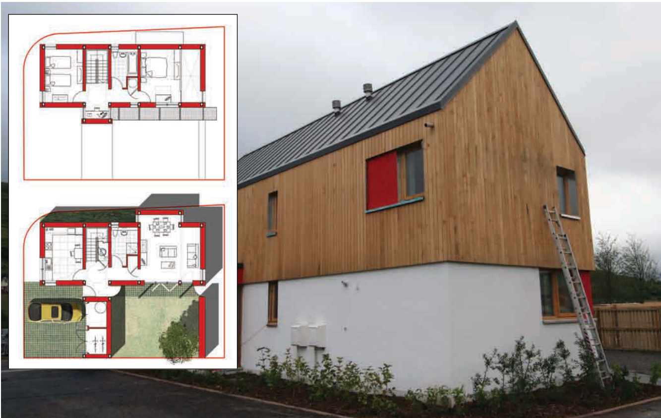
The Larch House, or 'Welsh Passive House' at Ebbw Vale is a certified Passivhaus, satisfying UK standards ENE 1,2 & 7. It achieved Code 6 of the Code for Sustainable Homes.
